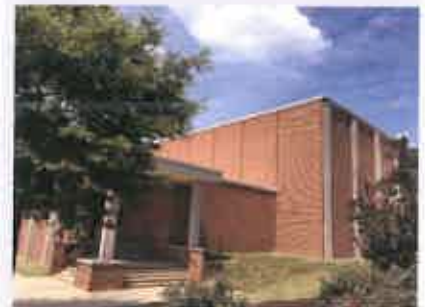
View of façade.
