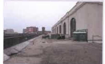
View of main roof area.
