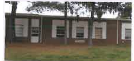
Partial view of existing windows and walls.
