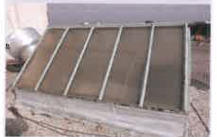
Existing skylights to be replaced throughout
