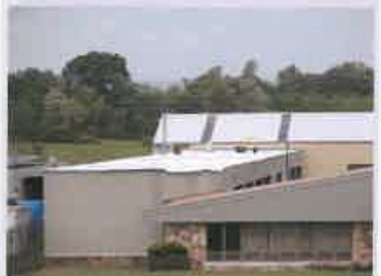
Single-ply replacement progress photo.
