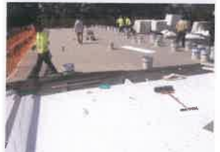
Installation of replacement roof system.
