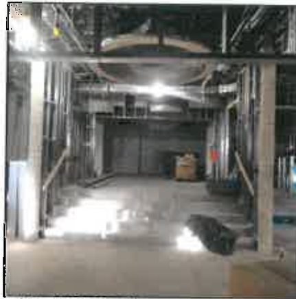
Lobby - In Construction
