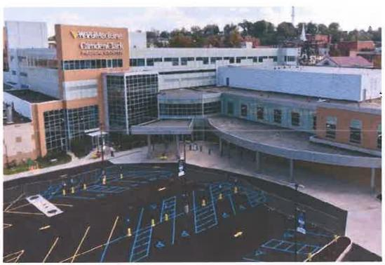
Camden Clark Medical Center hired Pickering Associates to reconstruct a portion of the hospital's North Tower Parking Lot. This project included transforming a former United Bank lot into a new parking section, as well as improving the overall flow of traffic throughout the hospital property and restructuring the parking layout. The team also coordinated with the West Virginia DOH to set up traffic flow patterns going in and out of the parking space.
