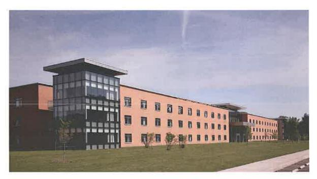
Security requirements for the command center influenced the design of the attached, copper-clad "black box" that is an homage to the native rock stratification seen throughout the state.
