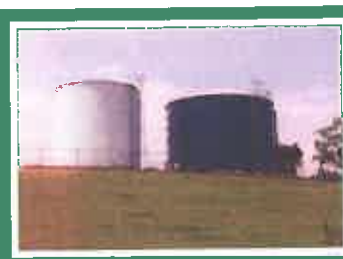
Alderson Water Storage Tanks
