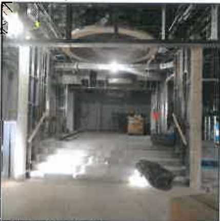
Lobby - In Construction
