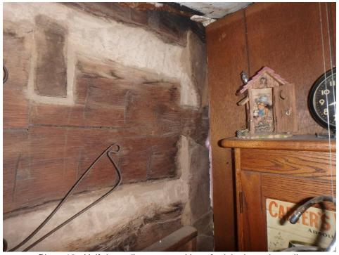
Photo 12. Half dovetail corner notching of original exterior wall.
