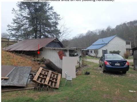
Photo 18. Left side view of root cellar 2, note modern front addition, cinder blocks replacing stacked stone (arrow), and house on right (looking south by southeast).
