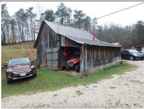
Photo 13. Front view of barn, note original exterior wall (left arrow) and side addition (right arrow) (looking north by northeast).
