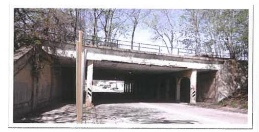
This project was a superstructure replacement of the Port Authority of Allegheny County East Busway over North Braddock Avenue Bridge. Markosky completed a Preliminary Design study to investigate the cost of using Accelerated Bridge Construction (ABC) techniques for this location and the Port Authority authorized the use of these techniques.
