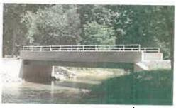
14'-0" wide. The superstructure of the replacement bridge consists of epoxy coated steel beams with custom designed precast panels and cast in place parapets. The abutments of the bridge are semi-integral abutments constructed of cast-in-place concrete. The bridge provides safe, high capacity access to a portion of the camp that would otherwise be isolated on the other side of the stream.
