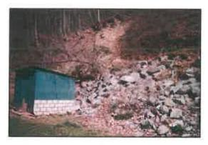
POTESTA prepared a regrading plan and design to re-stabilize the failed section of slide, including installing a new grouted riprap buttress, designing drainage at the toe of the buttress and around the existing residence, and restoring other problem drainage structures and areas that were installed as part of the original reclamation project. This work required the construction of a fence to protect the existing well house and adjacent occupied residence located on the site.
