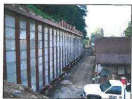
The retaining wall design required the application of a rock anchor tie-back system due to mine voids existing at the base of the hillside slope that were encountered during the subsurface exploration.
