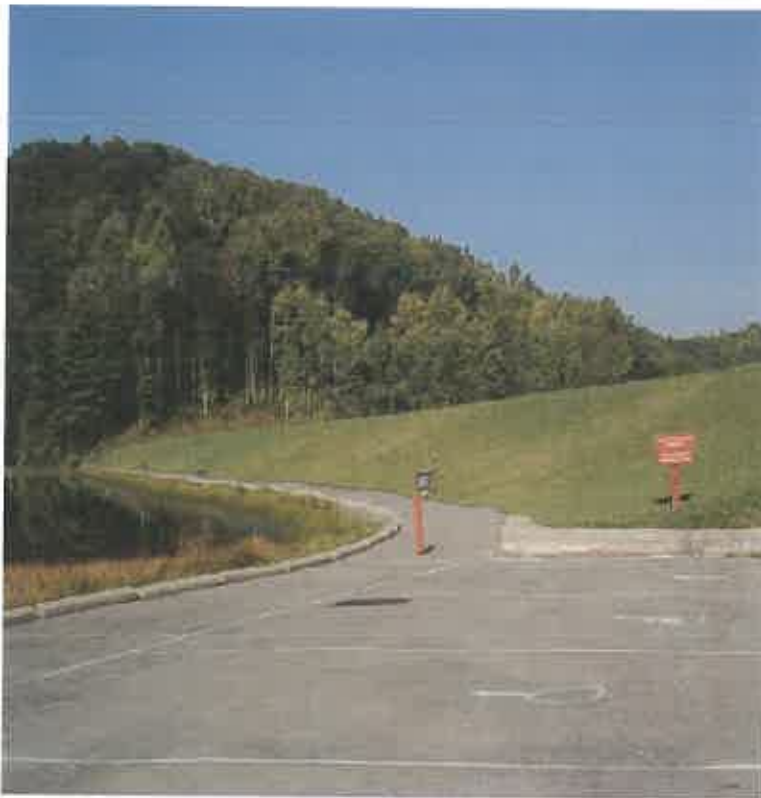
TETER CREEK DAM MODIFICATION, BARBOUR CO., WV
