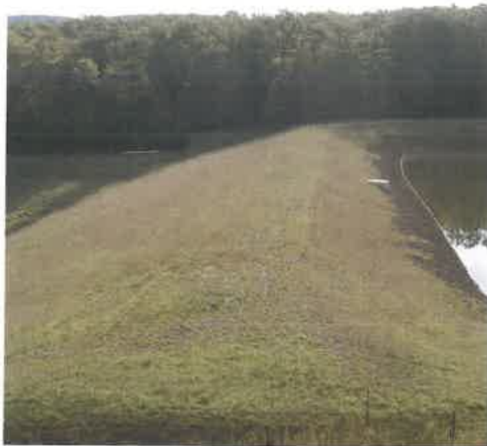
WILSON DAM MODIFICATION, HAMPSHIRE CO., WV
