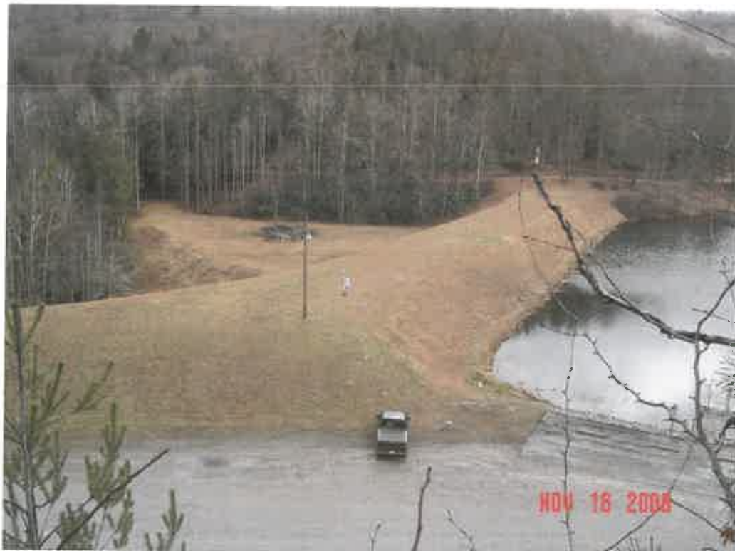
PLUM ORCHARD DAM MODIFICATION, FAYETTE CO., WV
