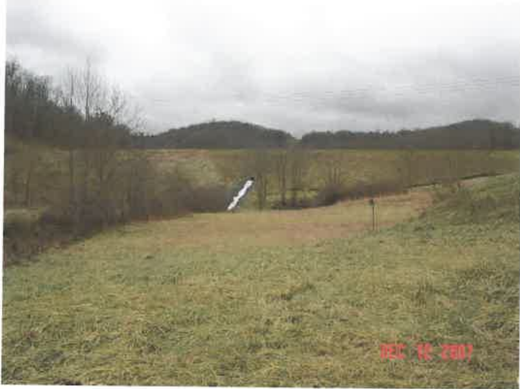
LEMLEY DAM MODIFICATION, MONONGALIA CO., WV
