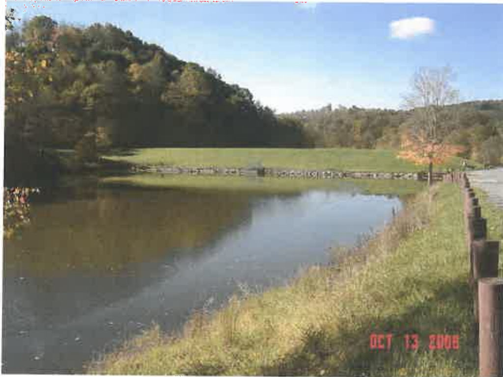
JIMMY LEWIS DAM MODIFICATION, MERCER CO., WV
