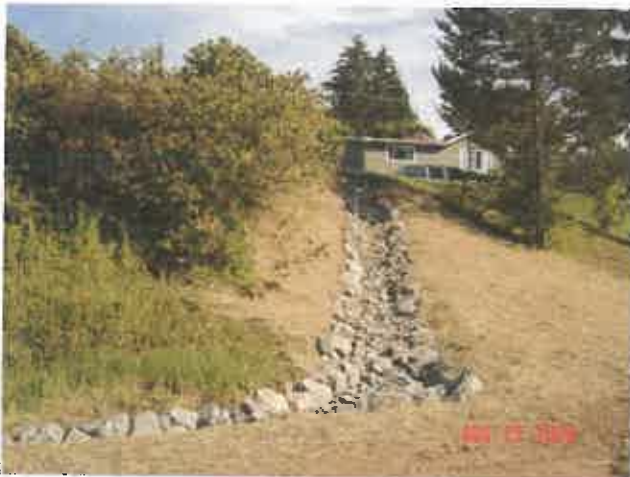
Erosion Repair – Rip Rap Armored Ditch
