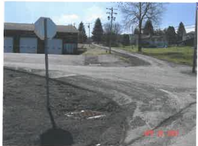
New Storm Drains and Catch Basins
