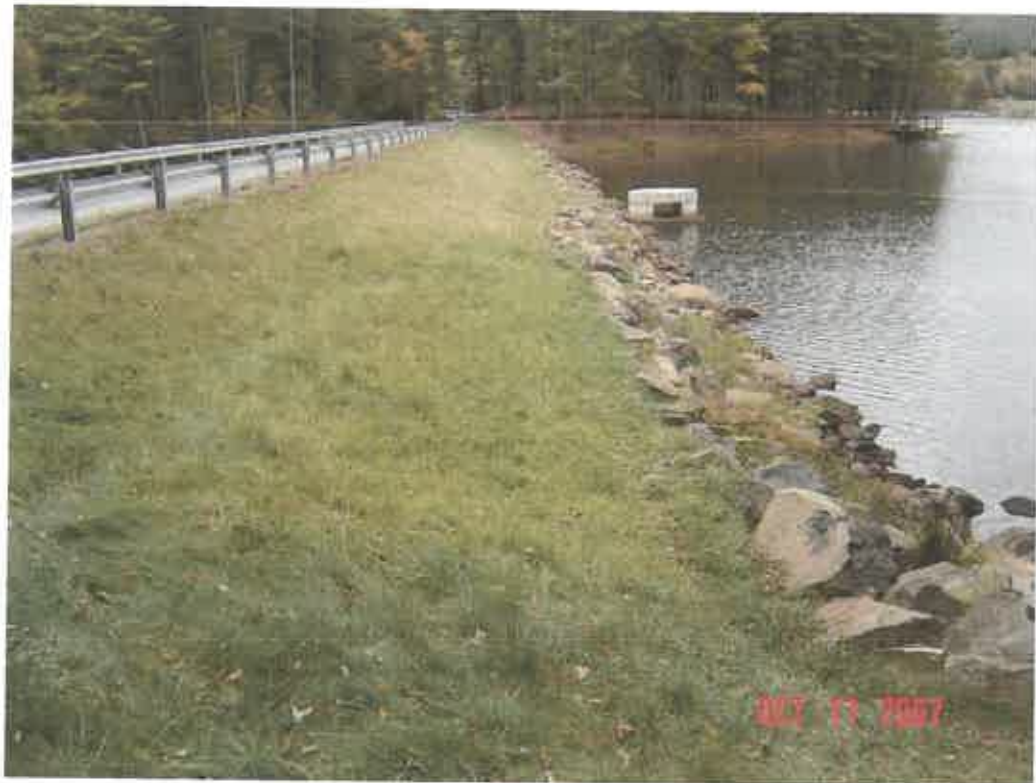
MONCOVE DAM MODIFICATION, MONROE CO., WV
