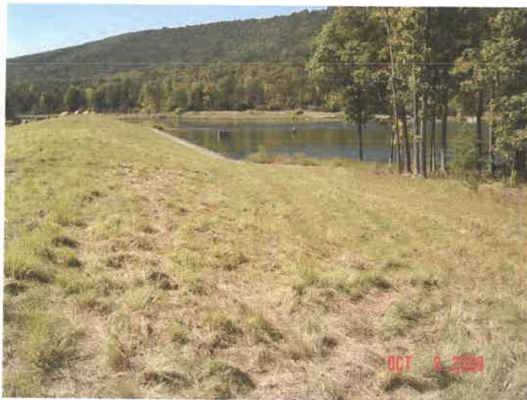
WARDEN LAKE DAM MODIFICATION, HARDY CO., WV
