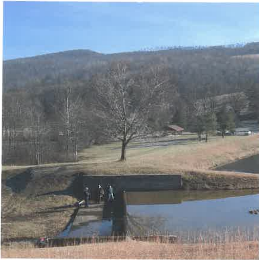
BELINGTON DAM MODIFICATION, BELINGTON, WV
