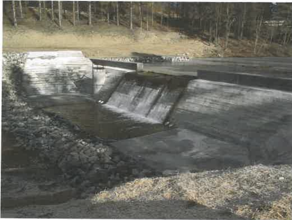
THOMAS DAM MODIFICATION, THOMAS, WV
