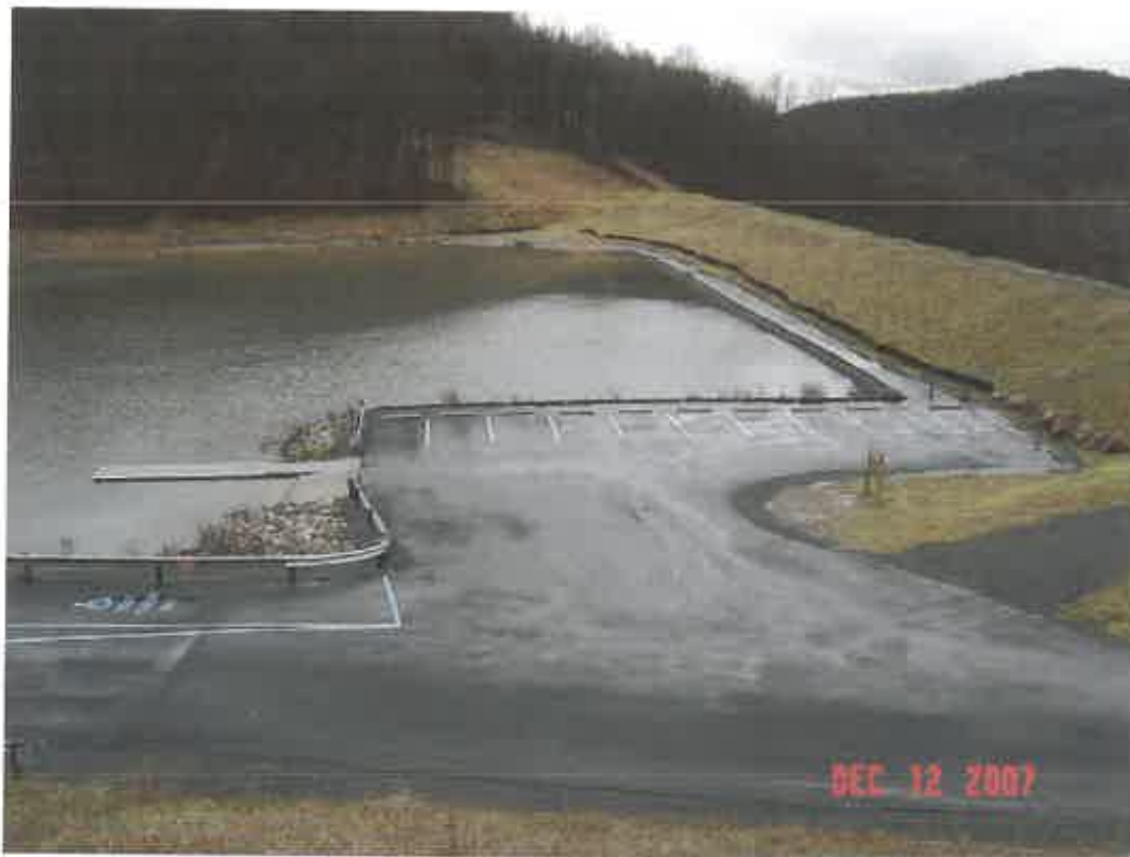
BAILEY DAM MODIFICATION, MONONGALIA CO., WV
