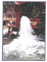
The "bubbler" borehole has an estimated flow of 500 gallons per minute (gpm). It had been cased and connected to a piping system for transport of the collected acid mine drainage to an existing passive treatment system. The borehole casing had been leaking for several years, and due to the artesian flow conditions, required replacement and abandonment to prevent direct discharges to the adjacent stream.
