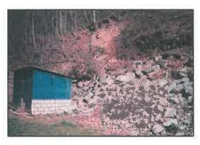
POTESTA prepared a regrading plan and design to re-stabilize the failed section of slide, including installing a new grouted riprap buttress, designing drainage at the toe of the buttress and around the existing residence, and restoring other problem drainage structures and areas that were installed as part of the original reclamation project. This work required the construction of a fence to protect the existing well house and adjacent occupied residence located on the site.
