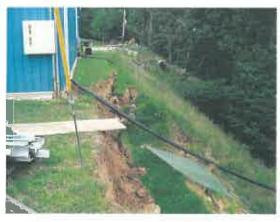
Potesta & Associates, Inc. (POTESTA) was retained by Columbia Natural Gas (Columbia) to evaluate and design remedial measures for a landslide at Columbia's Clendenin Compressor Station. The landslide was located adjacent to the office and maintenance building at the facility and threatened to damage the structure.
