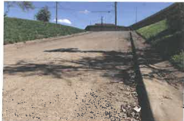
Existing concrete boat launch and concrete storm gutters
