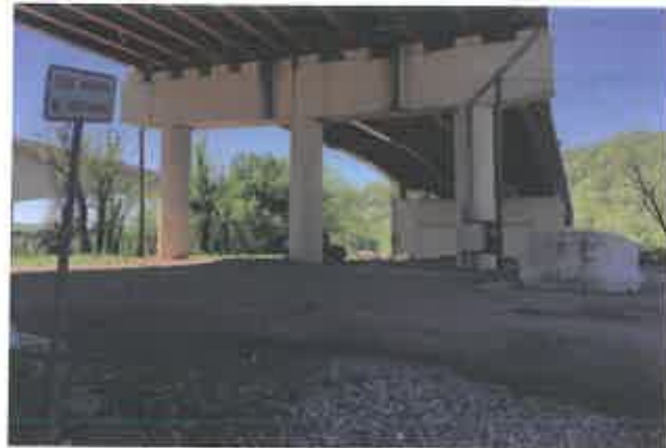
Existing gravel parking area under the I-64 westbound bridge.
