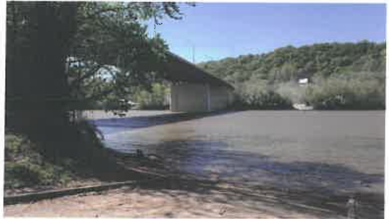
Bottom of existing boat ramp, looking downstream.
