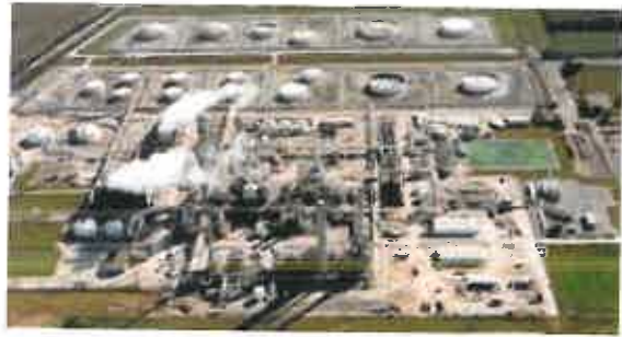
COSMAR Modernization Project Carville, LA
