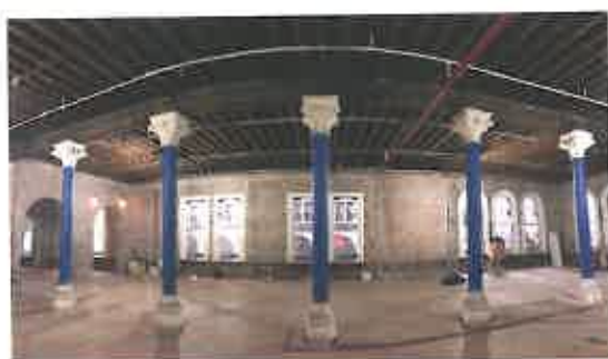
Floor Joist Assessment – Visual grading.
