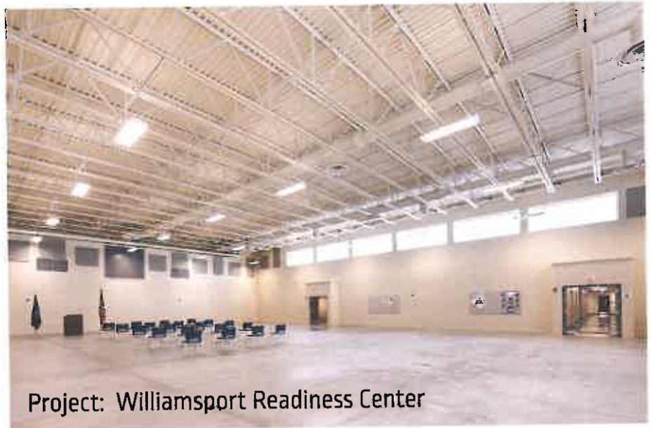
Project: Williamsport Readiness Center
