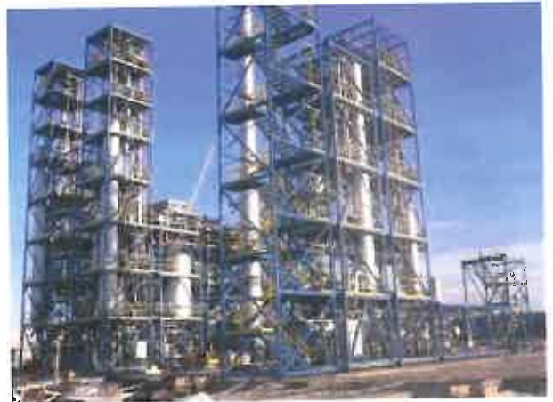
Polysilicon Production Facility Qujing, China
