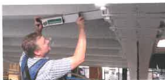
Resistograph testing of glulam arch.
