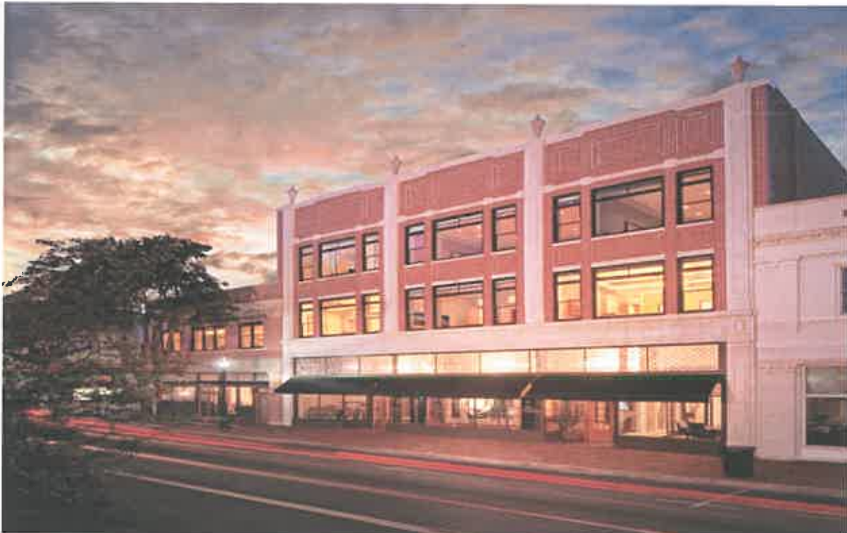
Thompson Headquarters, Sumter, South Carolina
