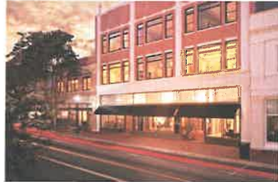
Corporate Headquarters, Sumter, SC
