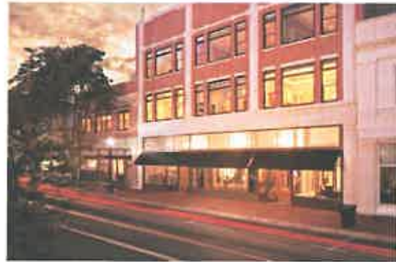
Corporate Headquarters, Sumter, SC
