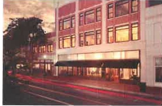
Corporate Headquarters, Sumter, SC
