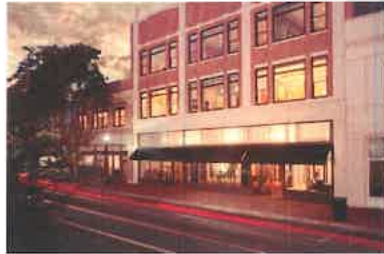
Corporate Headquarters, Sumter, SC
