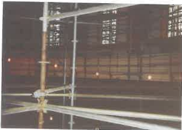
Photo during construction
