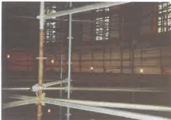
Photo during construction
