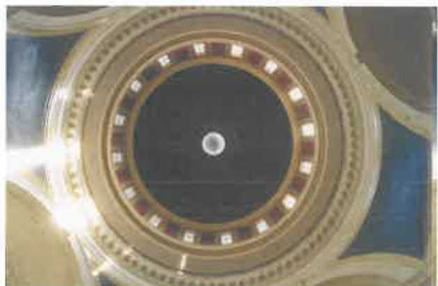
Photo of completed restoration
