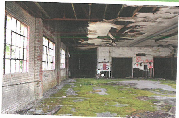
Right: Interior prior to renovation.
