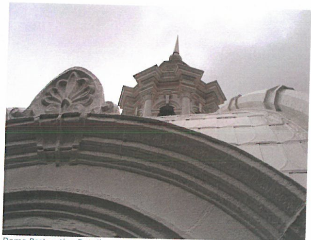
Dome Restoration Detail
