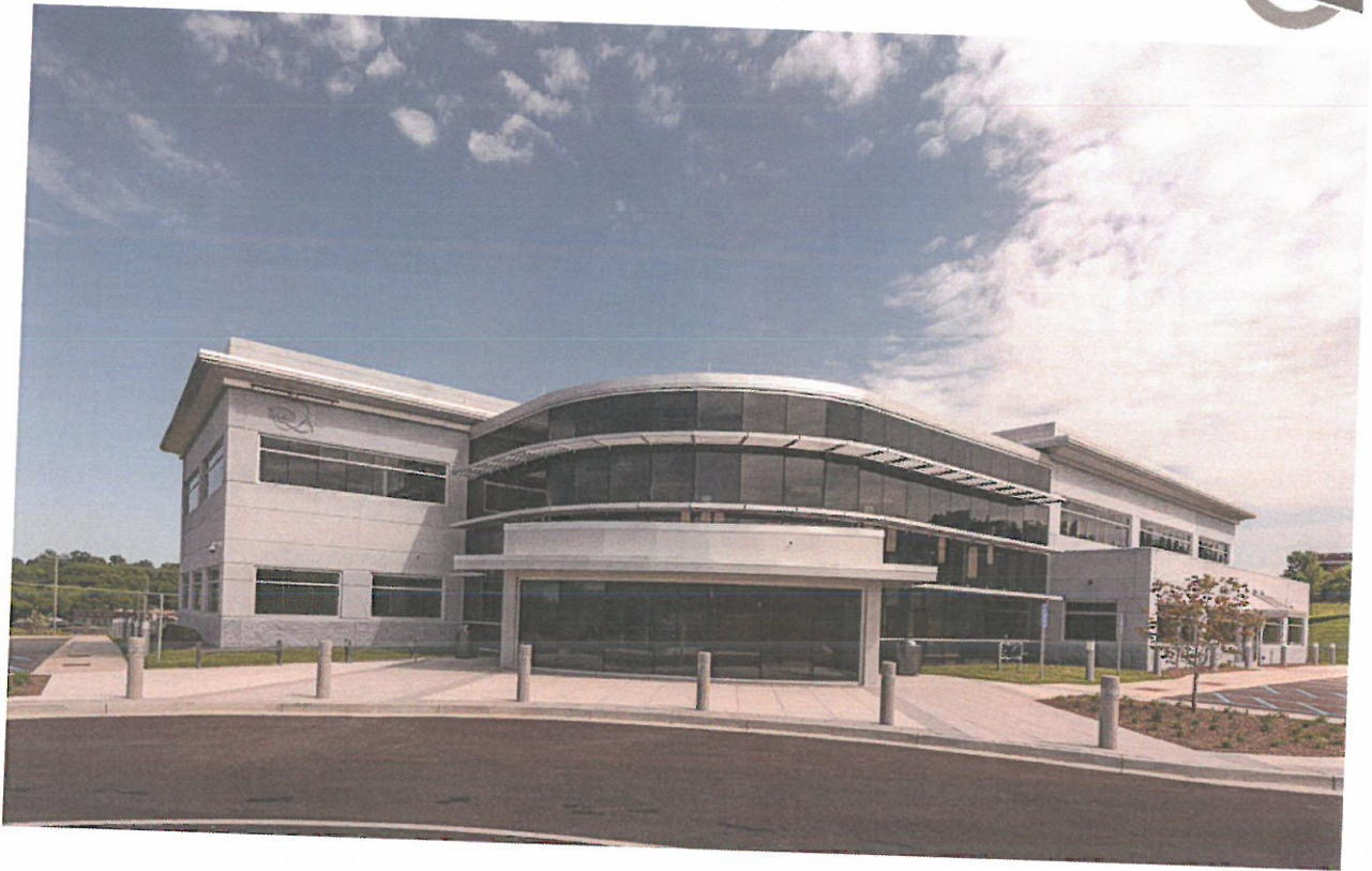
Frankfort Plant Board New Administration Building Frankfort, KY
