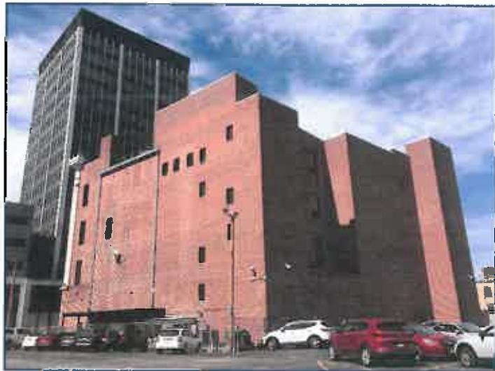
The back of the Revenue Center Building
