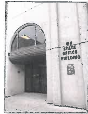
Beckley Building Entrance
