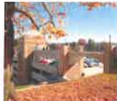
Fairmont State University Parking Garage Fairmont, WV
