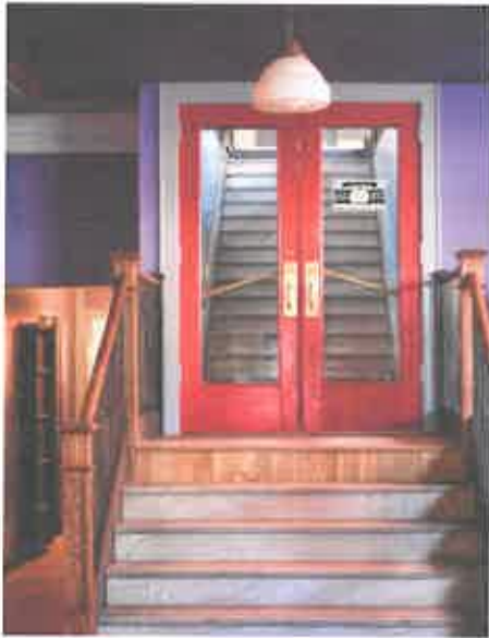
Uncovered stair from the 1920's found in the walls revived to match existing drawings
