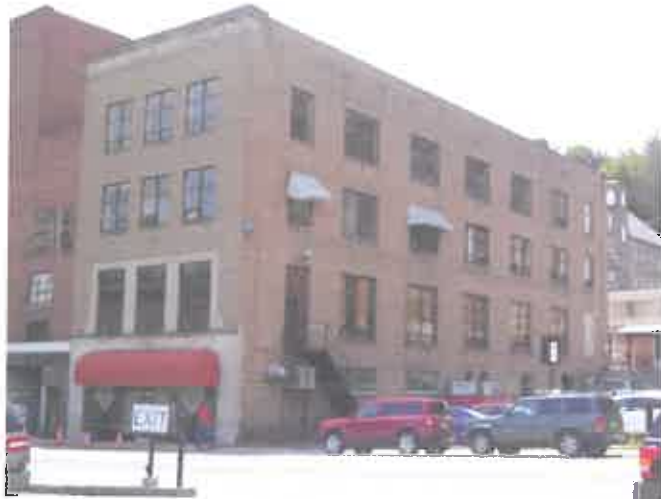
Existing Image (2014) of the AEP Building from Raleigh Street Bluefield, WV - Circa 1923 Architect Alex B. Mahood
