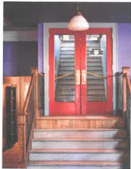
Uncovered stair from the 1920's found in the walls revived to match existing drawings
