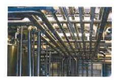
In a food processing facility, piping and conduit materials must be sanitary on the interior and exterior. We know the proper application of materials that are sanitary, able to withstand the abuse of chemical cleaning and hold up to temperature variations.
