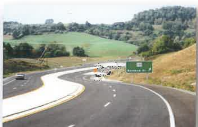
North Bridgeport Bypass
