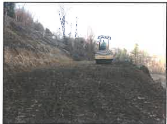
During Construction of Repair
