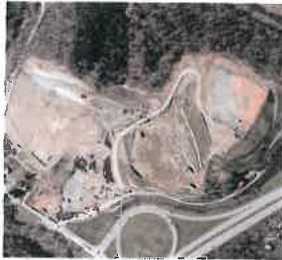
Gateway Development Site: I-79 Exit 155
