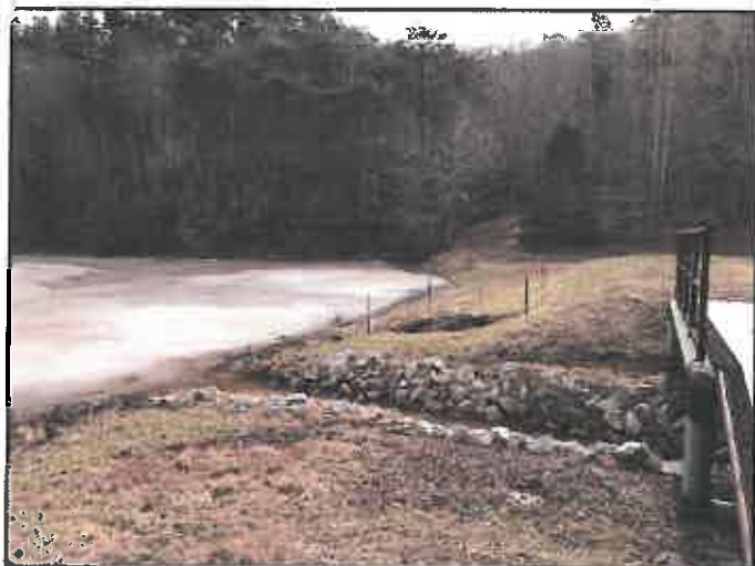
Cedar Lakes Dam No. 2
