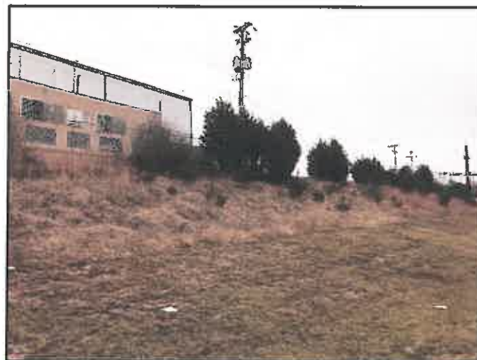
Slip Location at Food Distribution Warehouse
