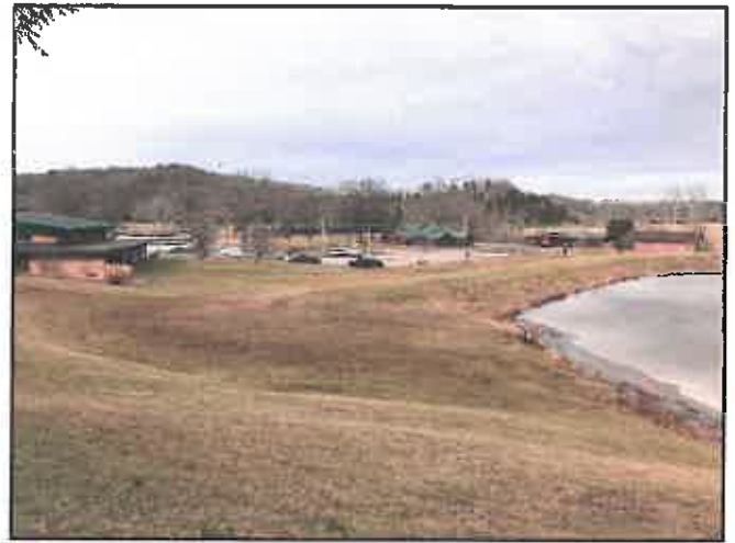
Auxiliary Spillway at Dam No. 1
