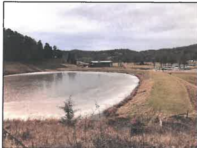
Cedar Lakes Dam No. 1
