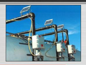
Direct-Injects's proprietary system offers reliable, solar powered diesel fuel improver injection.
