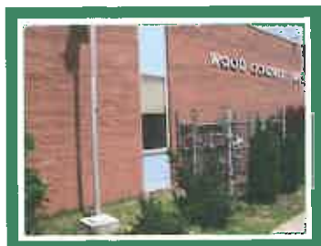
Parkersburg South High School
