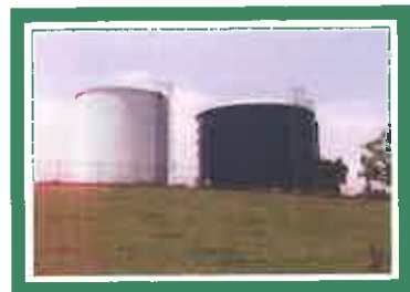
Alderson Water Storage Tanks
