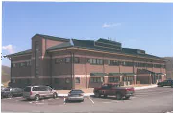
DISTRICT 6 OFFICE BLDG
