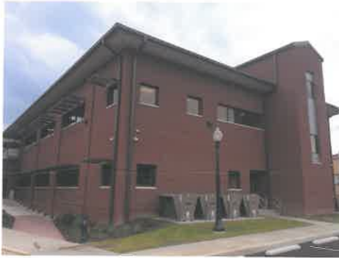
DISTRICT 1 OFFICE BLDG
