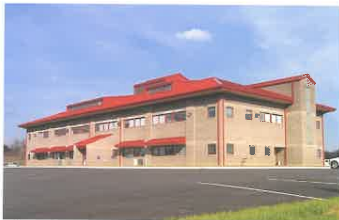
DISTRICT 10 OFFICE BLDG
