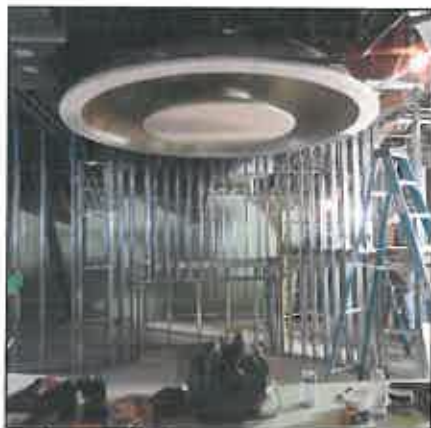
In - Progress Bar Area
