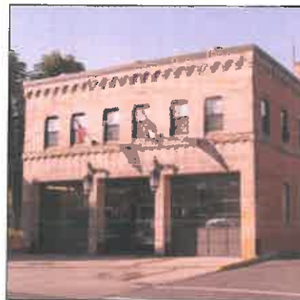
Central Fire Station
