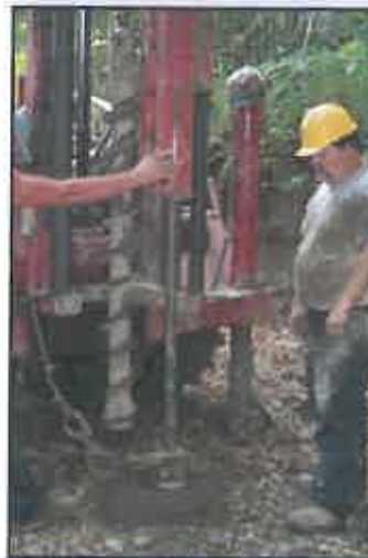
Drilling in Rough Terrain
