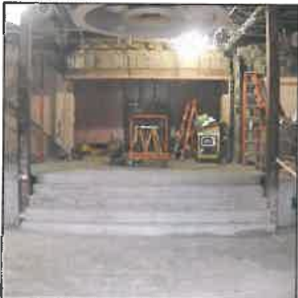
In - Progress Lobby
