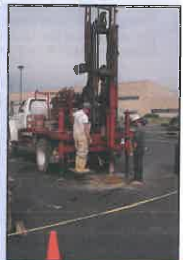
Drilling on Flat Terrain
