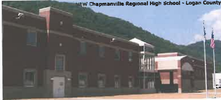
NEW Chapmanville Regional High School - Logan County
