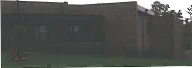
New Manchester Elementary School Addition/Renovations - Hancock County
