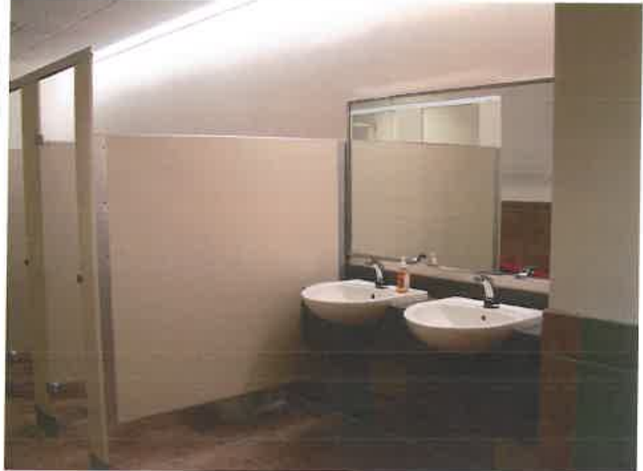
WVSP Detachment renovation
