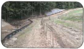
Burgess & Niple provided professional engineering services to the City of Newark, Ohio for their closed Watson Road Landfill. Repairs were necessary to meet the applicable surface water discharge limits within their NPDES permit for leachate discharge to a stream adjacent to the facility.
