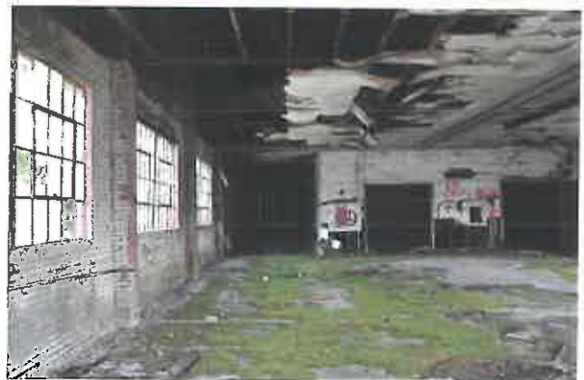
Right: Interior prior to renovation.
