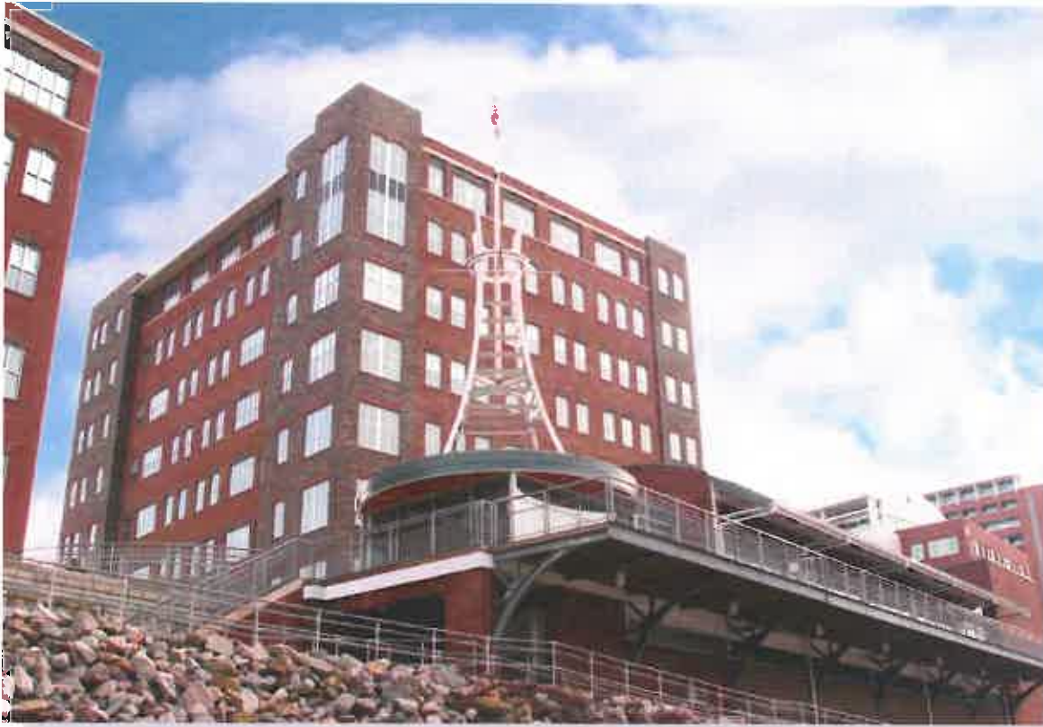
Marina Tower and Upper Monongahela River Center
