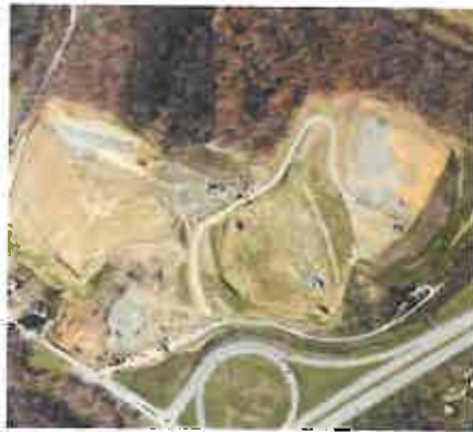
Gateway Development Site: I-79 Exit 155
