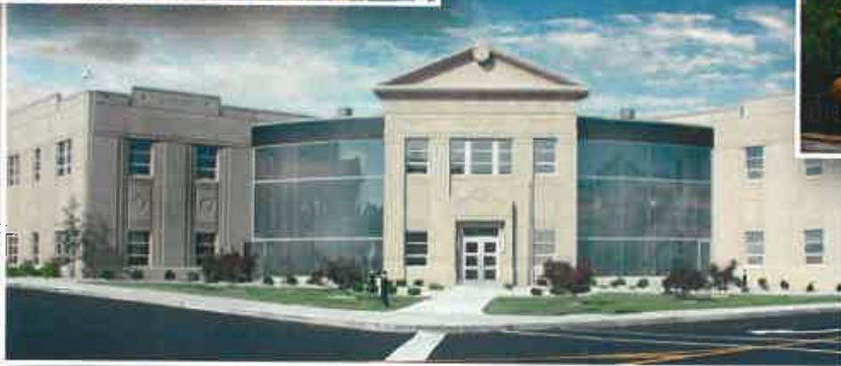
Mercer County Courthouse Annex
