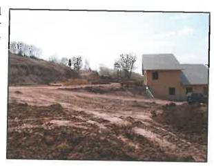
The fill locations were evaluated for geotechnical stability following the completion of test pits and borings. Project staff completed environmental permitting for the project including the preparation and submittal of NPDES construction stormwater permits and U.S. Army Corps of Engineers Section 404 permits.
