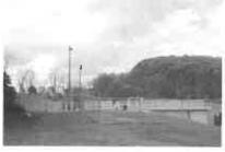
extended aeration wastewater treatment facility required to meet tertiary treatment effluent limitations complete with equalization basin, disinfection, effluent filters, mechanical head works, process control building, and an emergency generator. Extensive system evaluations were conducted to determine extent of Inflow and Infiltration
