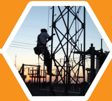
MICROWAVE/CELL SITE INSTALLATION & MAINTENANCE
