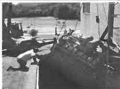
Crane lowering the emergency power generator into the electrical room.
