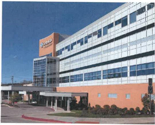
Camden Clark Medical Center contacted Pickering Associates to replace the windows in the North Tower on the Fourth Floor. The windows units were removed and replaced with new storefront windows with one inch insulated glass. These windows were similar in design to the windows for the Third Floor renovations that Pickering Associates designed. The windows incorporated new louvers for the PTAC units.
