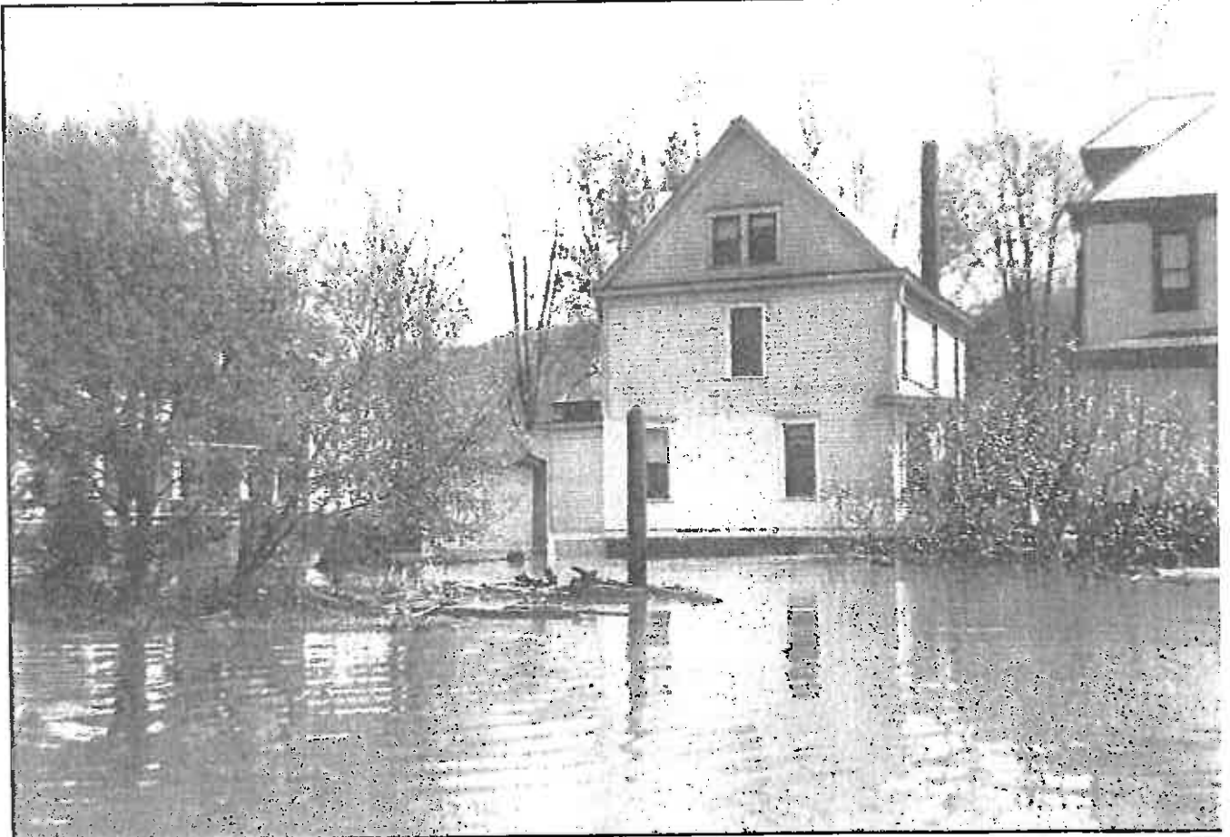
The back of our author's house with water filling the basement. During the worst of the floods, water would cover half of the first-floor windows.
