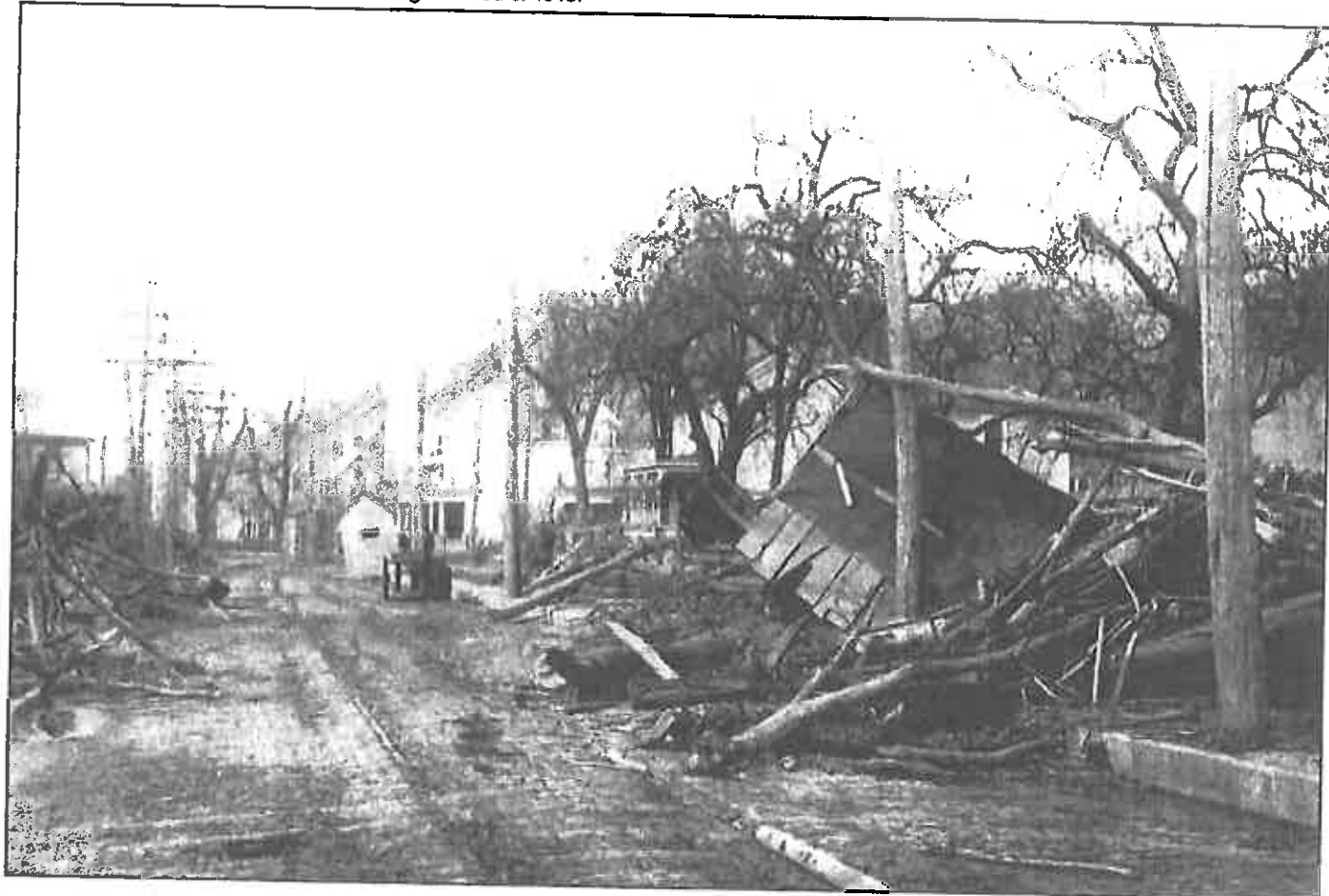
Maple Avenue piled up with debris following the flood of 1913.
