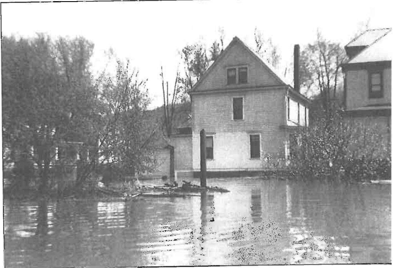
The back of our author's house with water filling the basement. During the worst of the floods, water would cover half of the first-floor windows.
