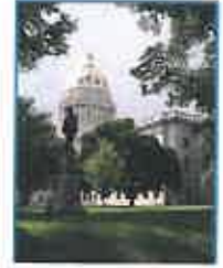
WV State Capitol Master Plan & Restroom Renovations
