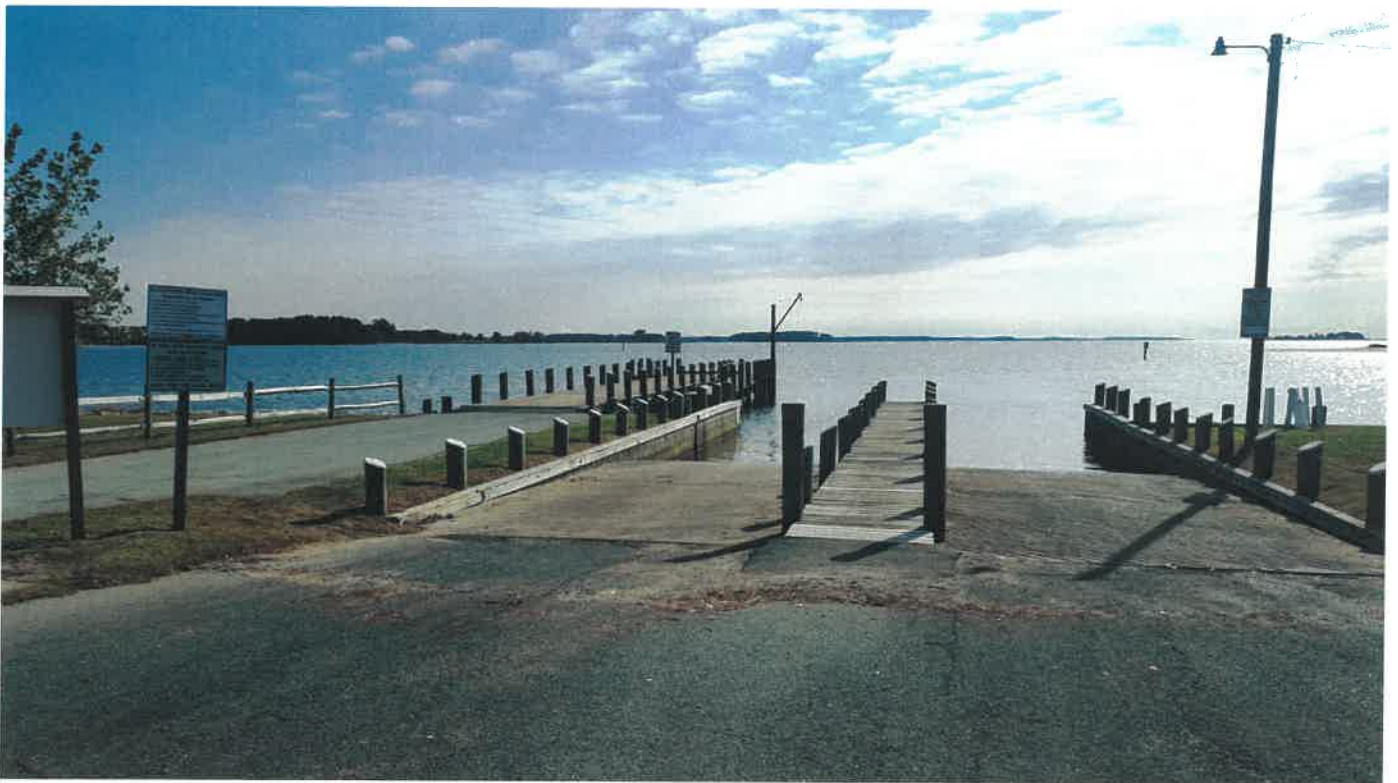
Piney Point Landing Boat Ramp and Pier
