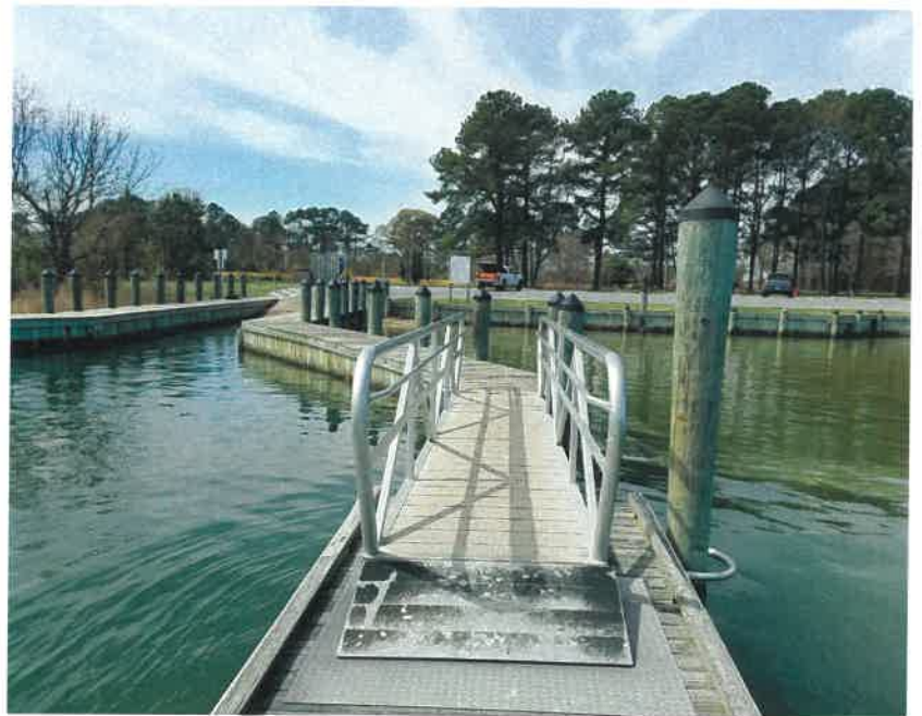
St. Inigoes Landing and Floating Dock
