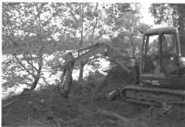
Monitoring of excavator creating trench to accommodate new boat docking facility.
